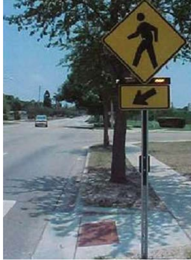
Figure 3: Rectangular Rapid Flashing Beacon (RRFP)
