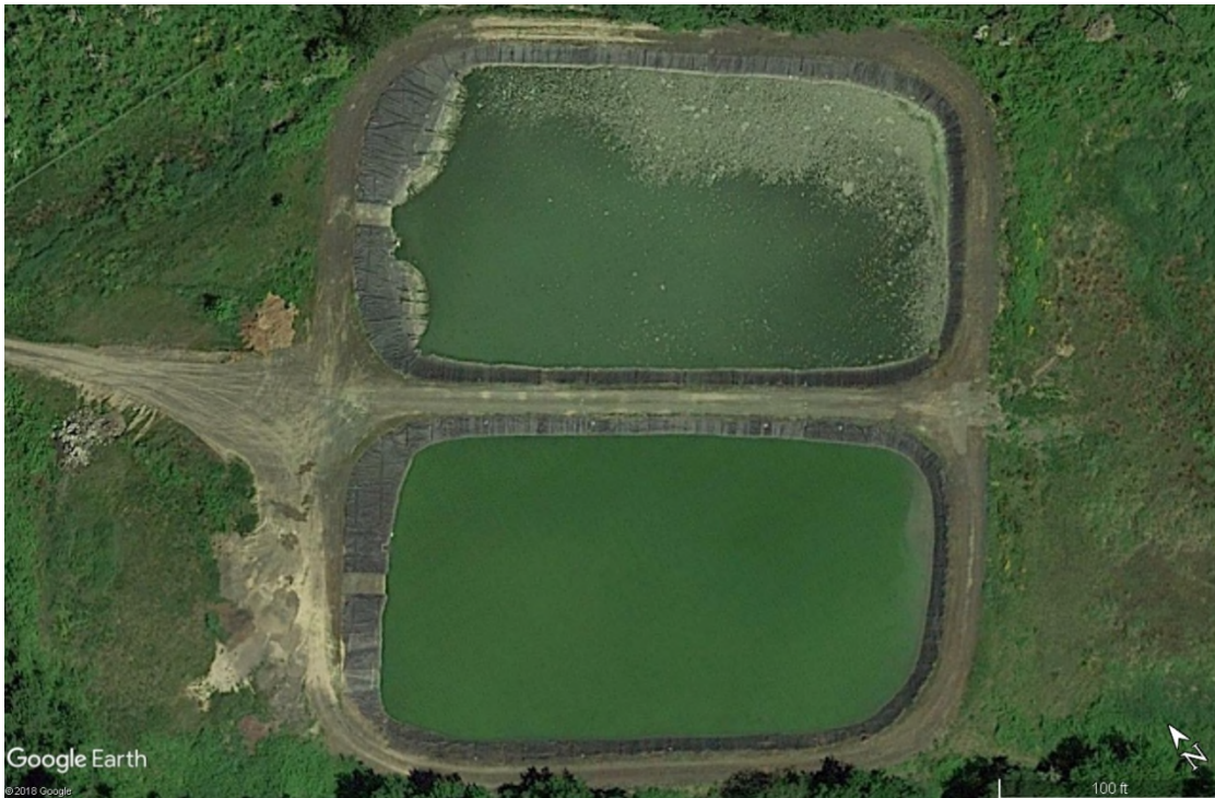
Figure 7-1. Lafayette STP Facultative Storage Lagoons
